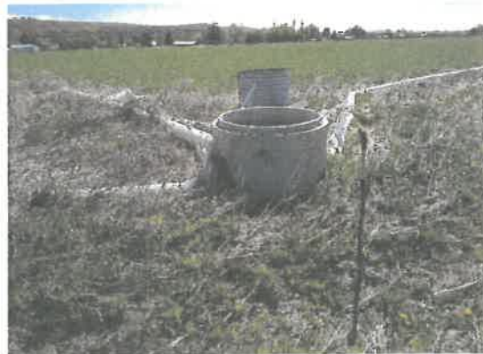
Photo 4 Irrigation weir and pipes. View toward E.
