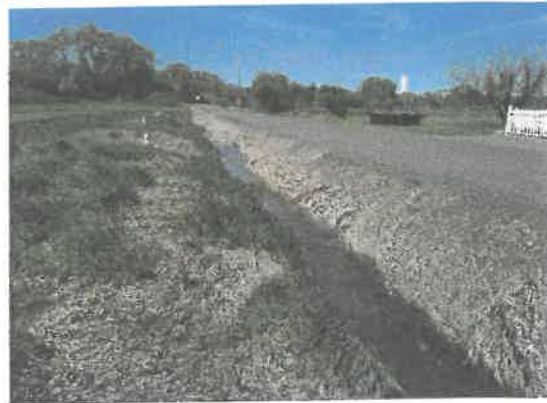
Photo 6 Type 2 (F) stream along Goodwin Rd. View toward W.
