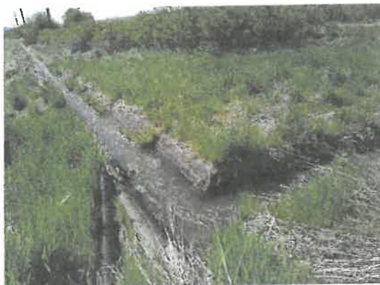
Photo 7 Gated concrete irrigation ditch. View toward S.
